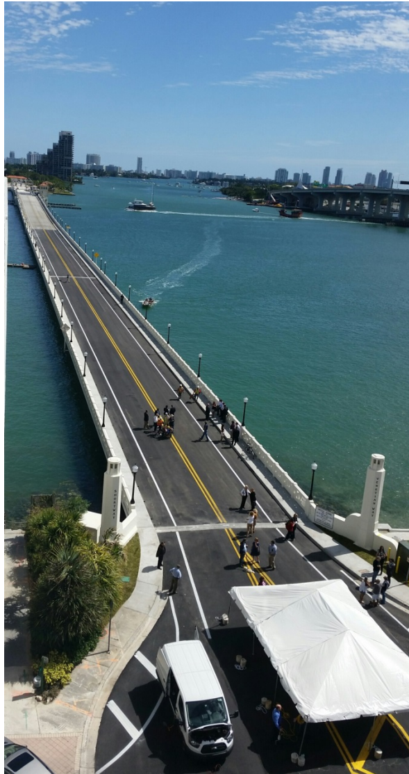
Venetian Causeway Bridge
